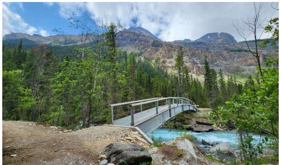
The new bridge at Whitehorn replacing the one damaged in 2021. /LAURA KEIL
