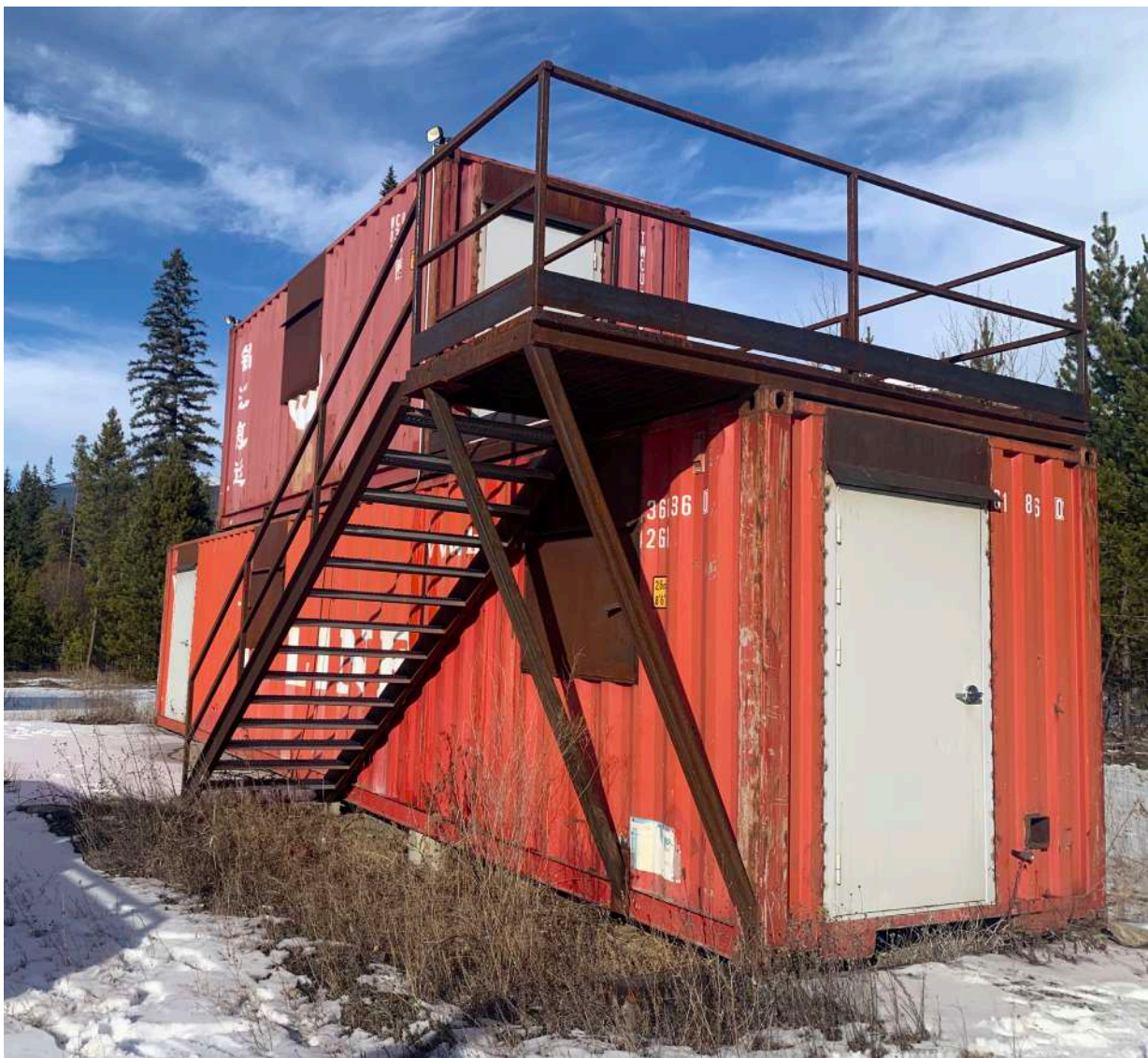
Constructed from shipping containers in 2016, Valemount’s live fire training centre will provide firefighters with hands-on experience in navigating house fires. The department will also install a freestanding door for forcible entry training. /ABIGAIL POPPLE
