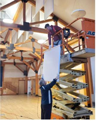
Tony Timotini hands up one of 60, 10lb sound baffles to Stephen Lance as they near the end of the installation at the McBride Community Centre. The new baffles will cut the reverberation time of noise by over half. This will provide event goers a clearer sound by eliminating most of the echo bouncing around the room. /ANDREA ARNOLD
