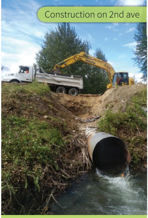
Crews are hard at work replacing the culvert on 2nd Ave in McBride. Once the culvert has been installed and the road returned to a drivable state, it will once again be open for public use. It has been over two years since that area of 2nd Ave has been open to vehicle traffic. / SUBMITTED
