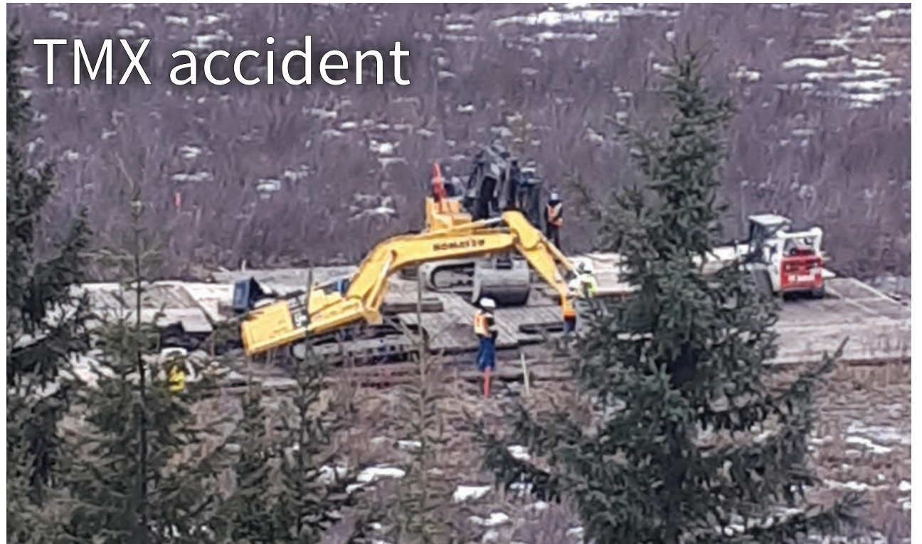
An excavator sank over a section of Trans Mountain pipeline in a swampy area just west of Jasper. A witness said they believed the workers had finished with a dig to inspect the old pipe and were removing the rig mats when one of the rig mats gave way. Trans Mountain did not confirm these details by presstime. The photographer said the company called in more equipment and rig mats on Monday to lift the machine off the pipe. The photo was taken on Hwy 16 just west of Jasper. /SUBMITTED
