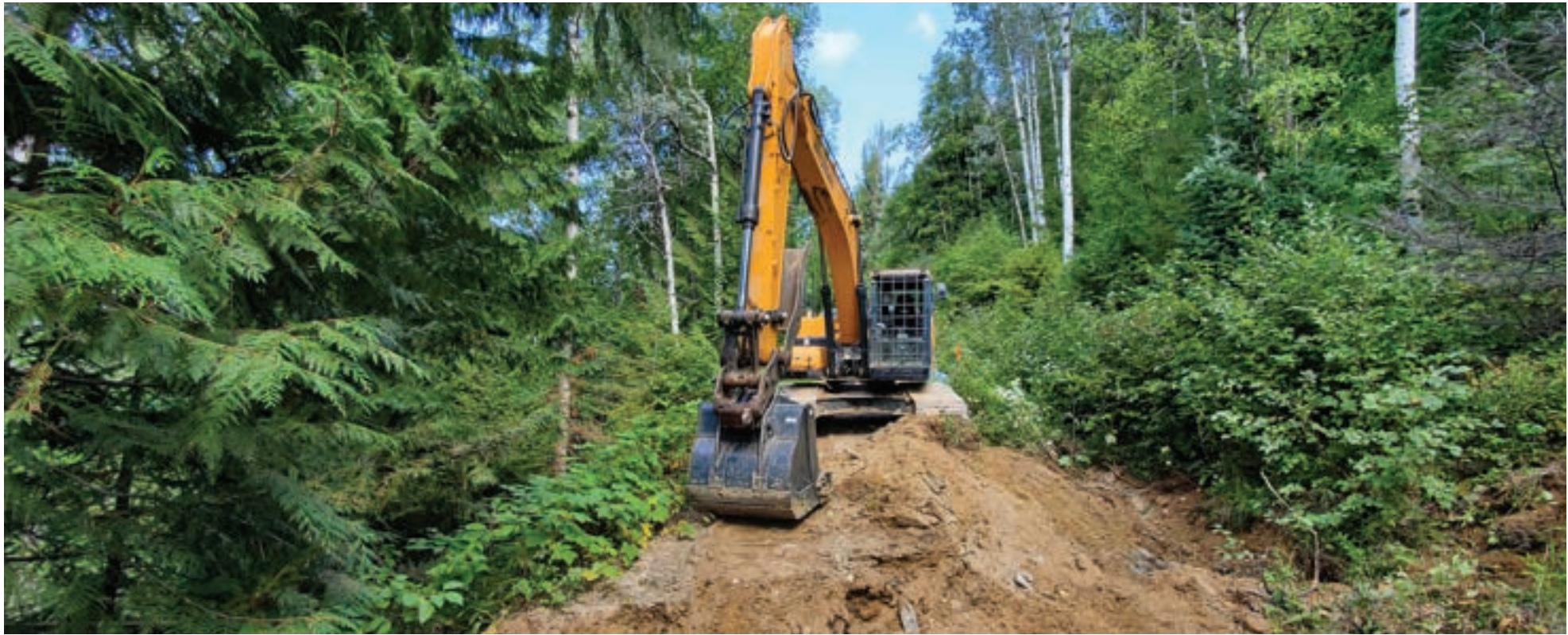
Site manager Chris White from Civil North Consulting is repairing and widening the road, and ditching as he makes his way up to the sluff at 6.5km, just below the McBride Peak halfway look out. He is also laying the many culverts that have been placed along the road. This work will help prevent erosion from the spring runoff. /ANDREA ARNOLD
