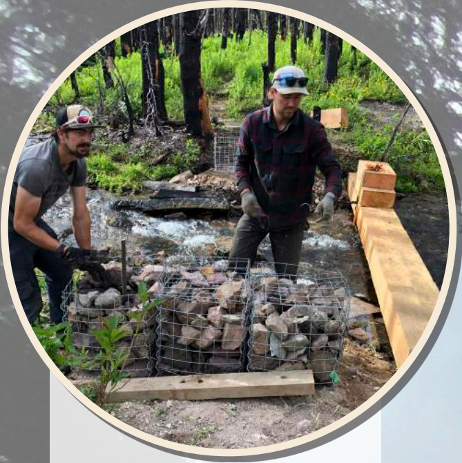
ABOVE: Sean Carson and Chris McGauley set up gabian baskets for bridge footings on the Akamina project in south east BC. /ANDREAS THONI
