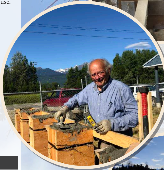
LEFT: Tom Jamin of "Thomas Jamin Woodworking" ensures the anchors are plumb in the footings for Akamina cabin. / ANDREAS THONI
